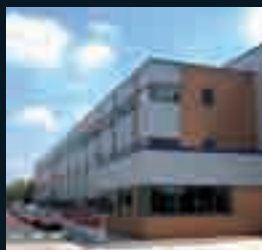
» US Gold was based in this building in Birmingham, where CentreSoft ran its distribution business
